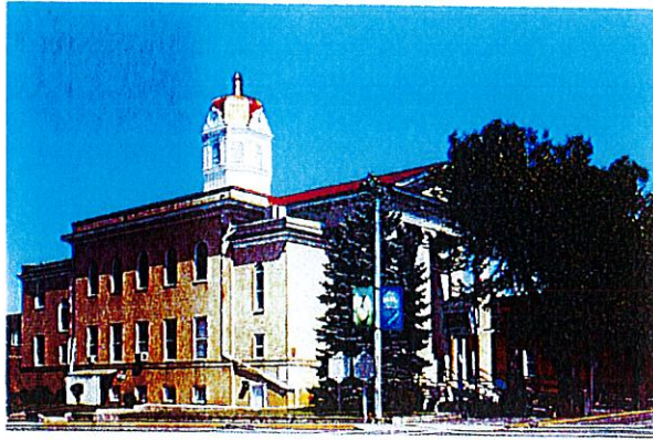
Hampshire County Courthouse, Romney, WV
